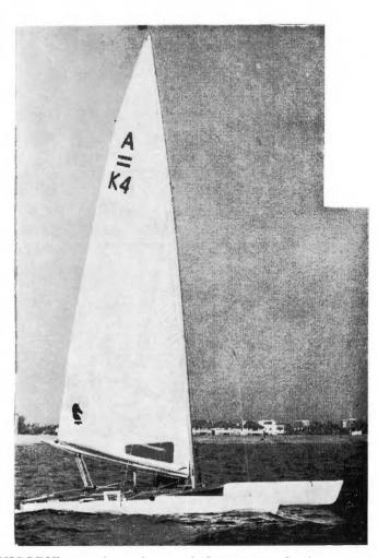
UNICORN's una rig carries a typical catamaran sheeting arrangement. A full width horse is fitted to the aft beam whilst a curved track is used for the kicking strap.
