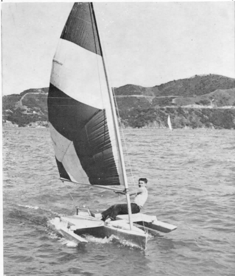
Arthur Piver's 12' fibreglass Trimaran with solid plastic foam floats
