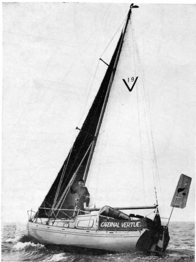
Dr. Lewis's single handled Transatlantic entry Cardinal Vertue had a vane operated trim tab that was really a part of the main rudder. 1960. (Photo: Eileen Ramsay)
