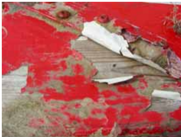
Peeling paint on the wooden float
